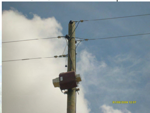
VROT-18-3R connected to RS232 port reads: I [A], U[V], W[kWh], [kVA]
