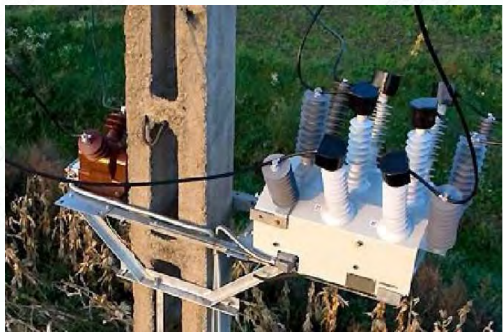
VTOP 2-27 PICTURE & EXAMPLE OF OUTDOOR INSTALLATION
